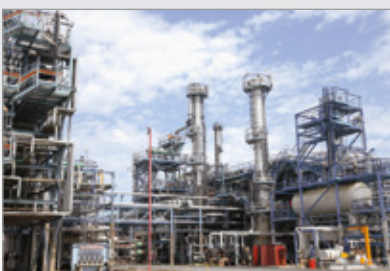
Refinery equipment (option)
